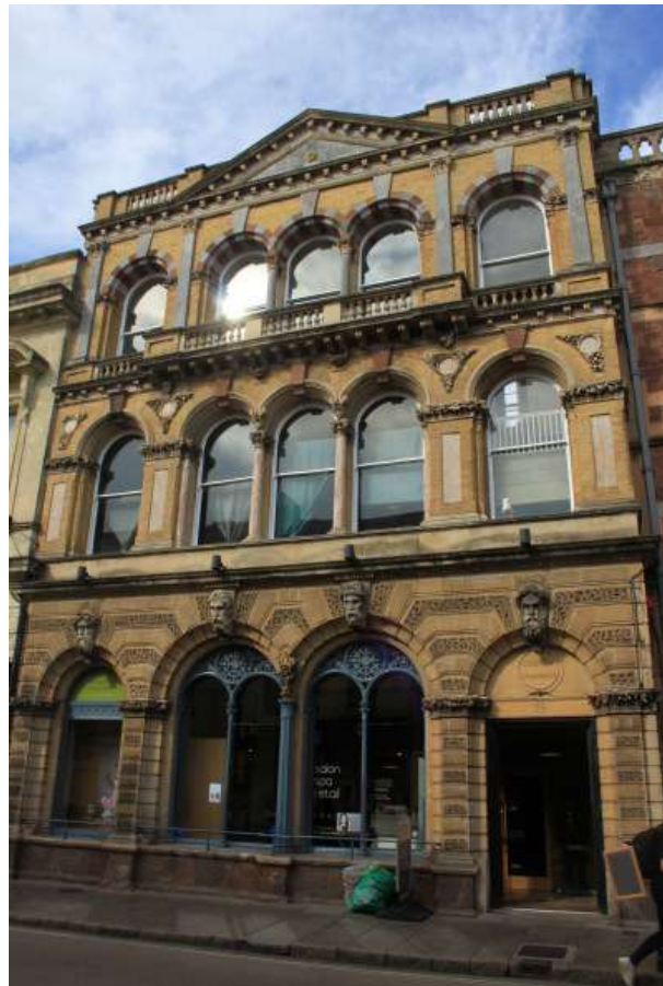
Figure 26. Detail of decorative cast iron in the ground floor windows of the County Chambers (below), with thanks to Estella Browne.
