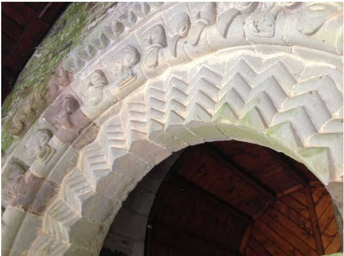
Figure 8. The inner order of chevron to the doorway at Buckland Brewer. Note the projecting points of each voussoir.
