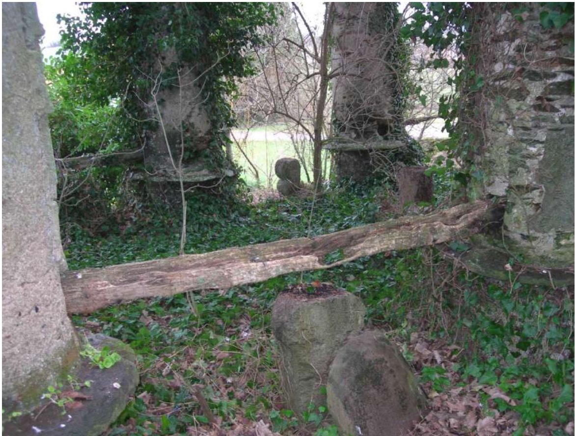
Figure 7. A surviving floor rail with block A and its fallen staddle beneath it.
