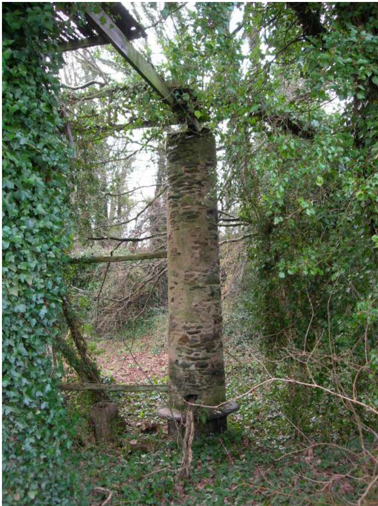
Figure 9. The north-west column with linking floor rails but no mortice for an intermediate rail at this end of the barn.
