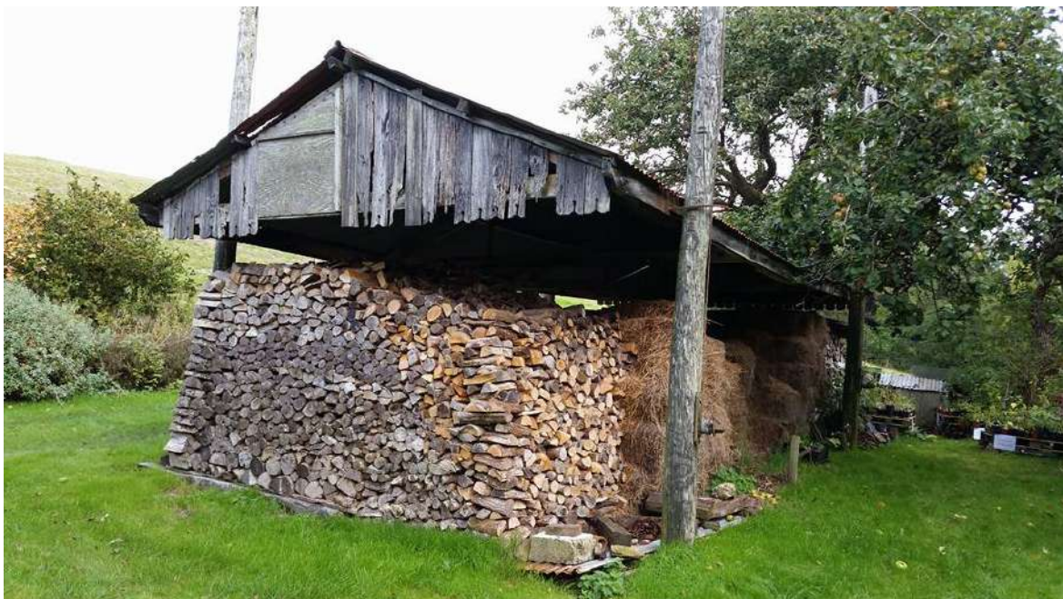
Intriguing 'Dutch' barn at Bridge Mill, repaired with telegraph poles.
