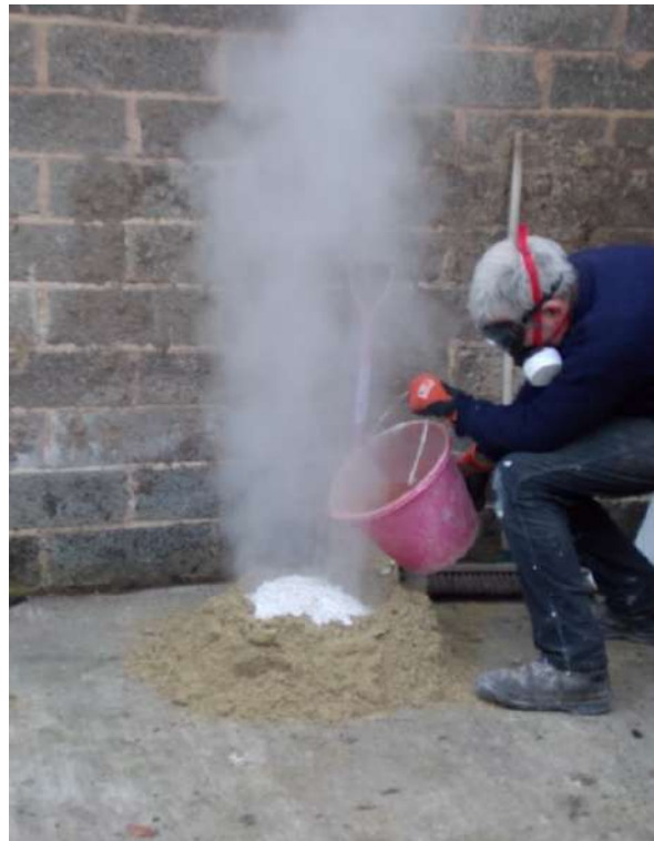
Above left. David Tyler demonstrating slaking lime. The quick lime is first added to water already in the tank, this photo was taken as additional water is added, as the initial quantity of water boils away.
