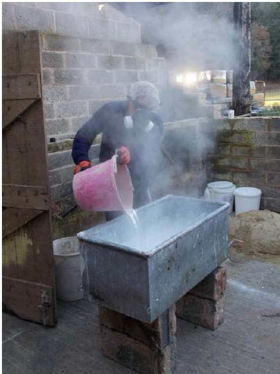
Above left. David Tyler demonstrating slaking lime. The quick lime is first added to water already in the tank, this photo was taken as additional water is added, as the initial quantity of water boils away.
