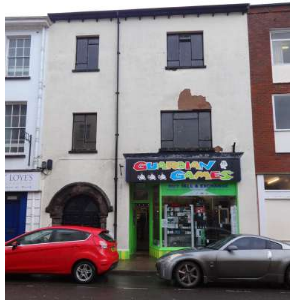
No 27 Bampton Street, Tiverton in December 2017. The ground floor is currently tenanted by Guardian Games and the building appears to be poorly maintained.
