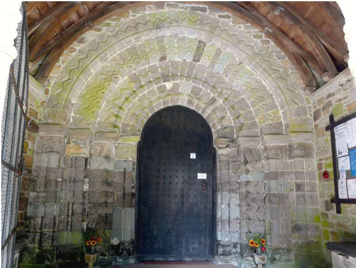
Figure 13a. The south door at St James, Kilkhampton.
