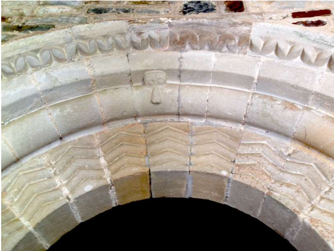
Figure 9. Detail of the doorway at Parkham to show the single beakhead in the centre of the arch.
