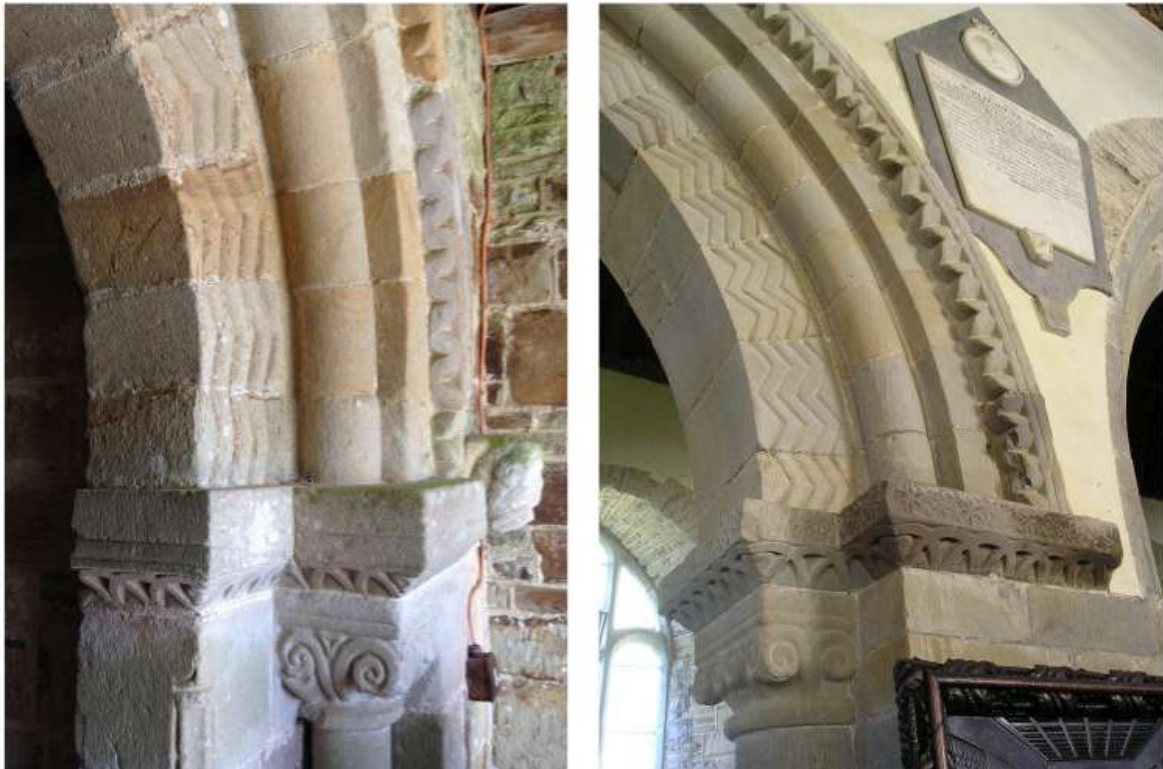
Figure 10. The near identical decorative schemes to the south door at Parkham ( left ) and the easternmost arch of the north nave arcade at Morwenstow ( right ).
