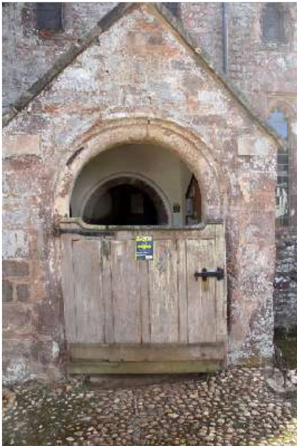
Fig. 5. A half-door to the outer doorway of the porch at the church of St Mary, Poltimore. This is an uncommon survival, probably late 18th or 19th century, although the outer doorways of porches often preserve evidence of fixings.
