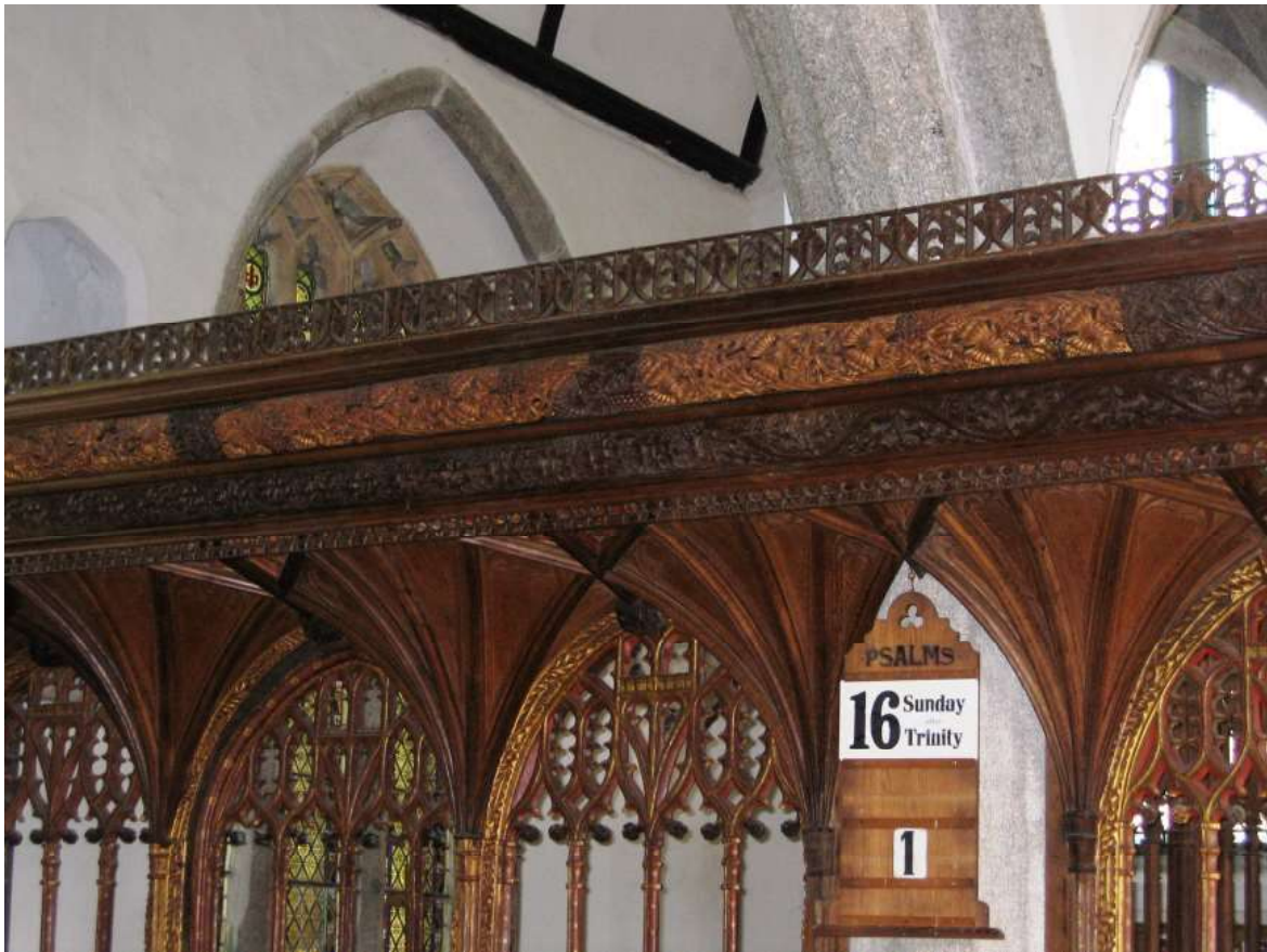
Fig. 2. The restored 16th century screen at Manaton (1890), showing the gilded original carving and the ungilded Pinwill work.
