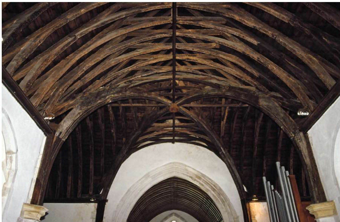
Fig. 7. The roof of the crossing of the church of St Mary, Luppitt.
