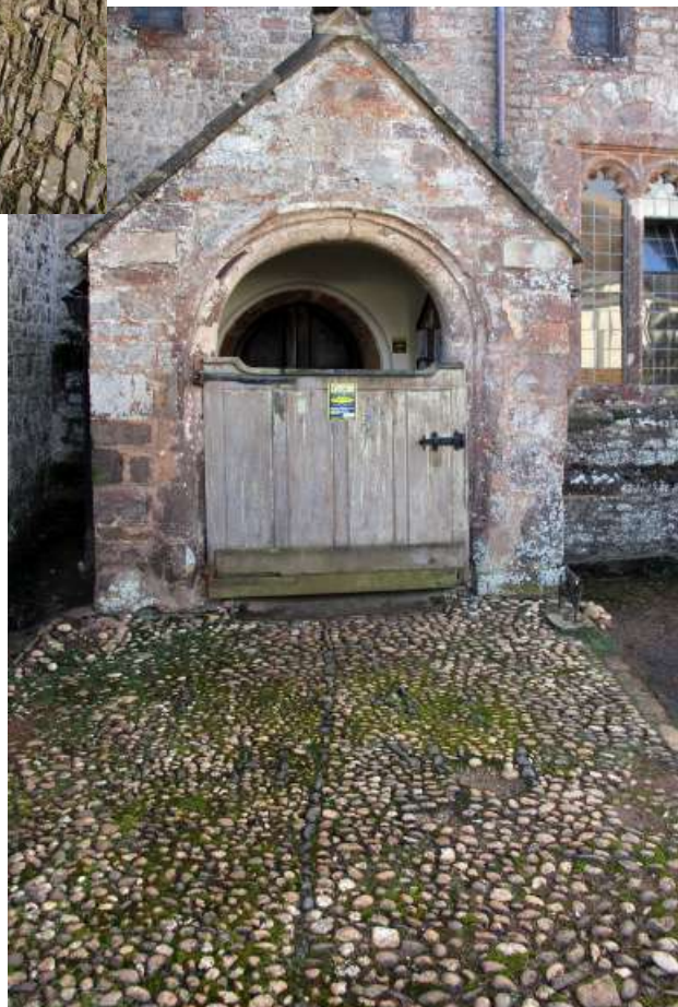
The church of St Mary, Poltimore, has a random laid path of small, rounded cobbles (right). This has a spine of dark grey cobbles and includes the date 1743 and initials (detail, below).
