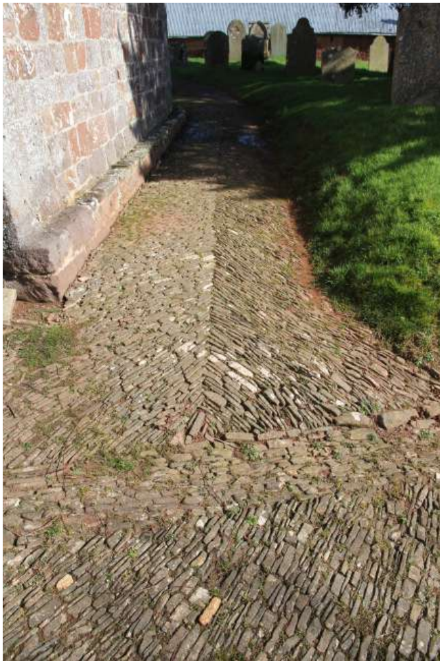
One of the paths at St Andrew, Colebrooke, is herringbone, but without a spine (left).
