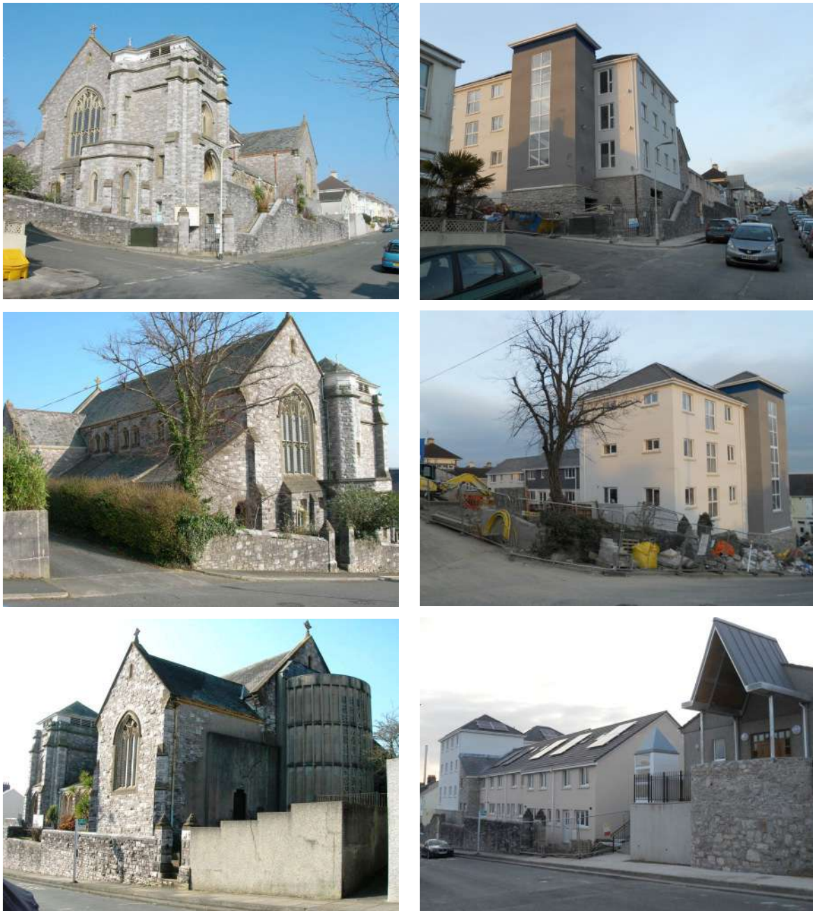
Fig.2. Views of the exterior of St Philip, Weston Mill, before and after demolition in 2014: (a) & (b) (top), from the south-west; (c) & (d) (middle) from the north west; (e) & (f) (bottom); before views 1.iii.2012, by Peter Child; ‘after’ views 22.iii.15 by Stuart Blaylock.
