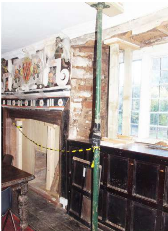
Above left. The condition of the hall stack and ceiling putting the 1605 overmantel at risk. Above right. The hall overmantel cleaned and secured.
