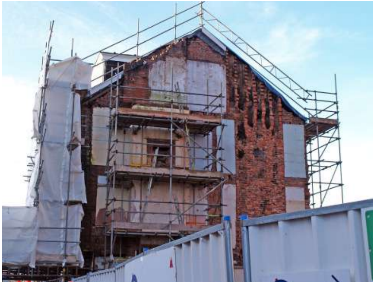
Fig.5. 5a) [Top left] The demolished stacks had a string course and cornice. 5b) [Bottom left] The shafts above the roofline were demolished because they were said to be dangerous. The internal shafts were scraped out by the contractors. Why? 5c) [Top right] The contrast between the lost stacks and their replacement is a microcosm of what has been lost in the development – proportion, detail, patina, elegance texture.
