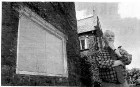
■ POOR IMPRESSION: Philip King by the boarded-up windows of the Grade I listed building, The Walronds
