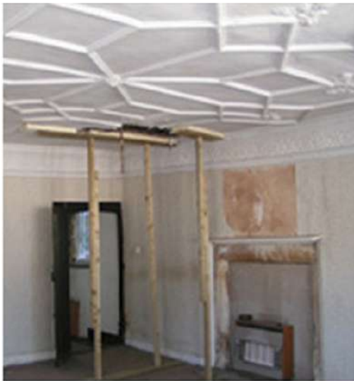
Ornamental plasterwork, propped to prevent collapse of ceiling [above left] and following repairs [above right].
