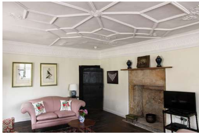
Ornamental plasterwork, propped to prevent collapse of ceiling [above left] and following repairs [above right].
