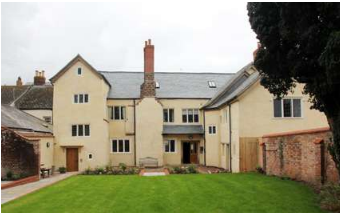
Rear elevation. Above. Perilous condition of the stair turret and the hall chimney shaft dismantled. Below. Following repair and rendering, the rear turret and chimney rebuilt, the chimney shaft reinstated and the garden redesigned
