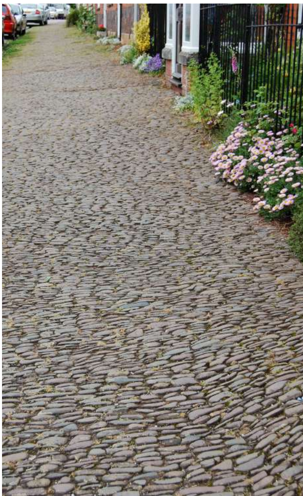
Fig.14. A raised pavement at Thorverton. Peter Marlow.
