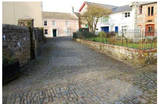
Fig.16. A cobbled roadway and pavement at Chulmleigh. Peter Marlow.
