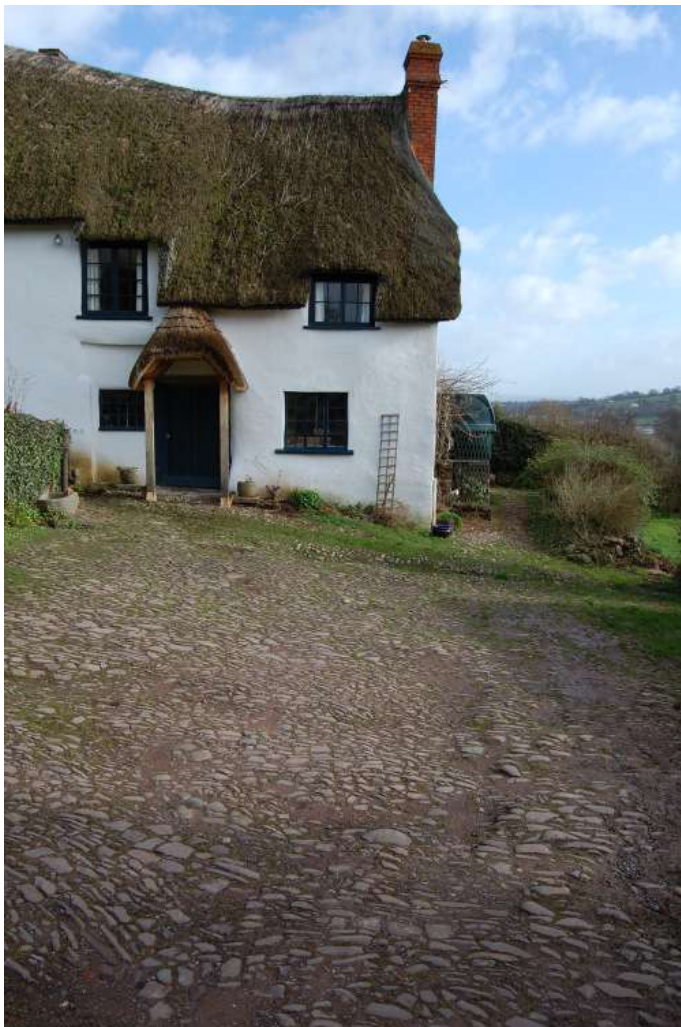
Fig.18. The yard at Gotham Farm, Tiverton. Peter Marlow.
