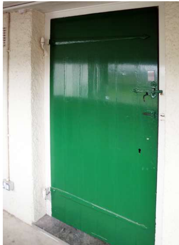
Fig.24. A door to the service wing rooms. Keystone, 2012.
