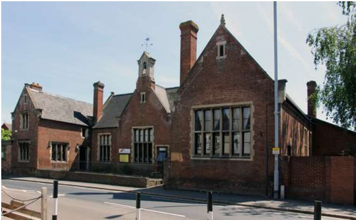
Fig.1. Cowick Street First School, Exeter. The DBG asked for this to be listed as part of our efforts to save some historic school buildings in Exeter. It was rejected for statutory protection on the grounds that it was too altered, but is on the local list which affords it some protection.
