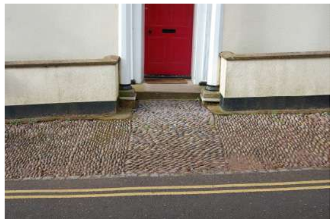
Fig.15. A nice detail at East Budleigh: an apron of beach pebbles laid at right angles to those of the pavement. Peter Marlow.
