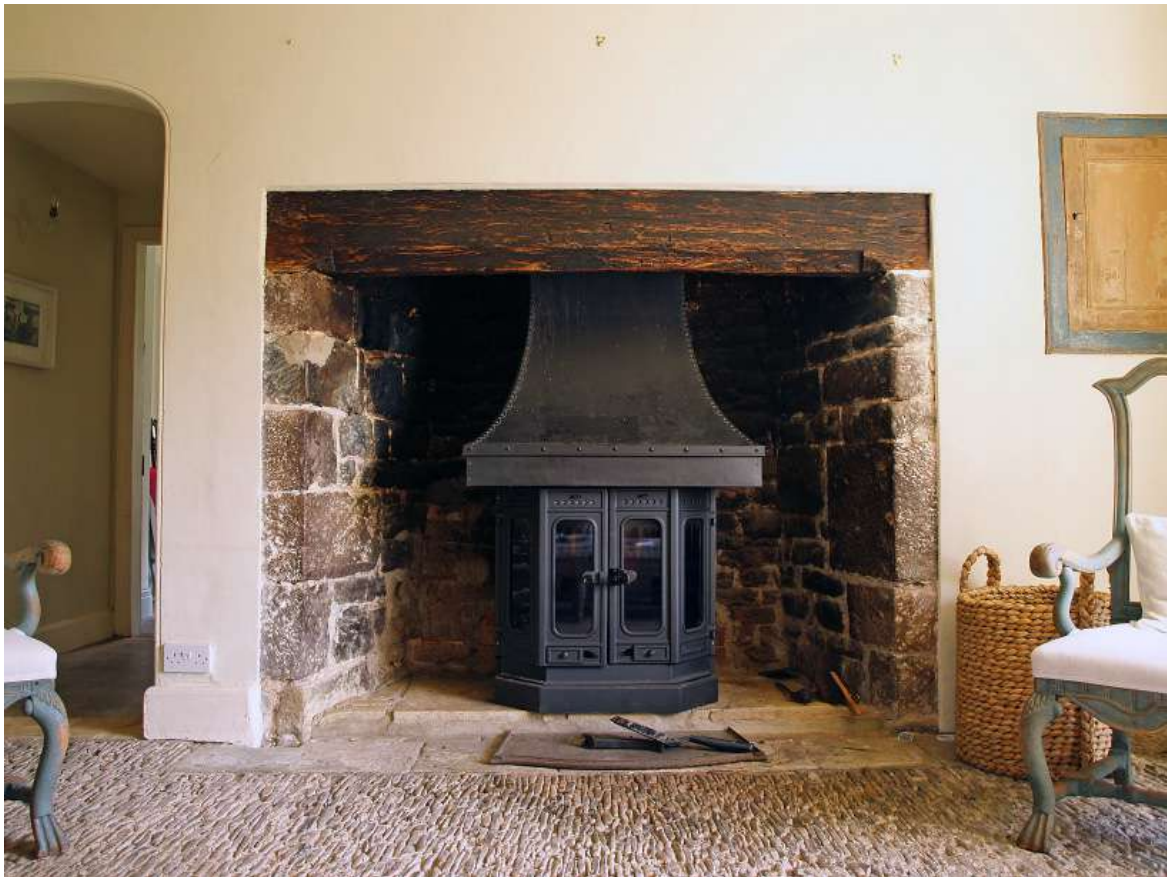
Fig.22. A cobbled floor to a good quality 17th-century parlour in a mid Devon house. J R L Thorp.
