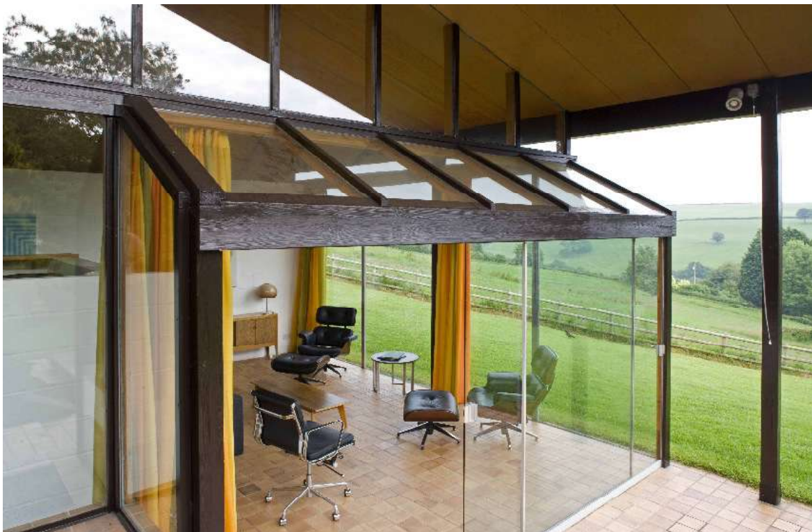
Fig.6. The roof appears to float over the building through the use of a 'clerestory' above the living area.
