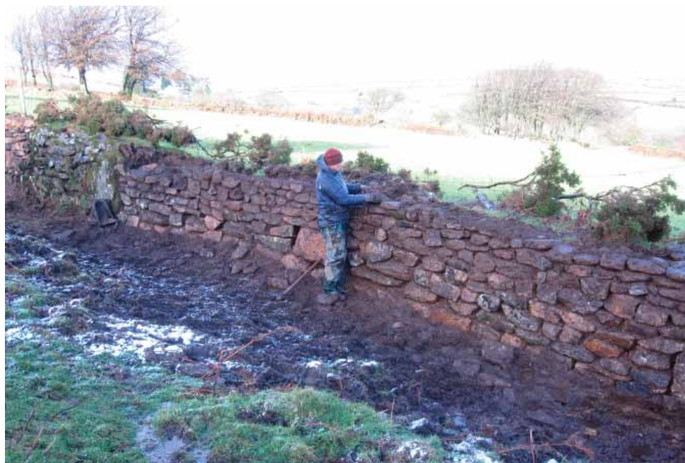
Fig. 7. Edward Vickers at work. Note the un-repaired section to the left. Here the ditch is yet to be cleaned out and the inner bank re-formed.
