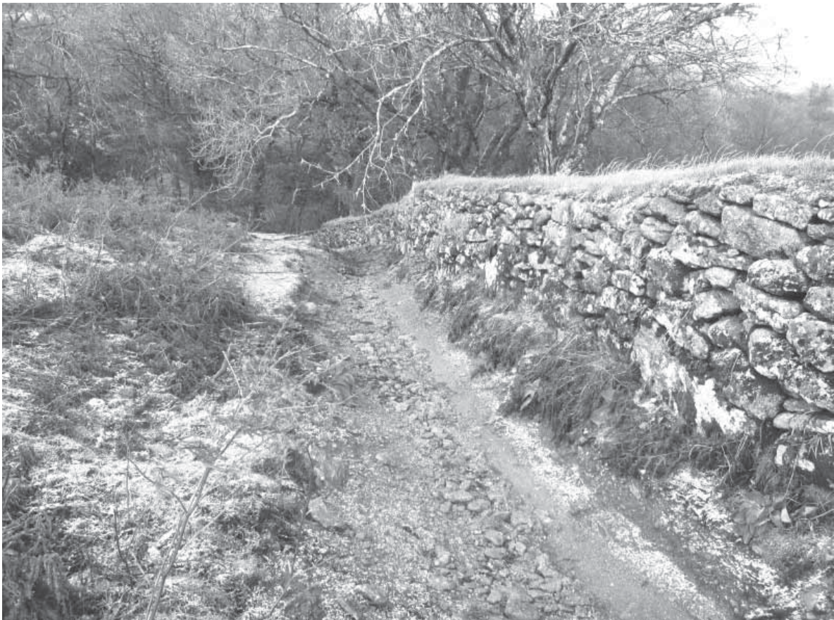
Fig. 4. Section CD1, Moorland side, looking downslope towards West Coombe.
