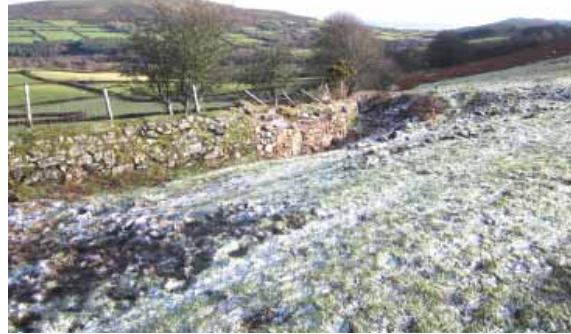
Fig. 6. Work in progress: Note the un-repaired section on left, old fence on top of bank, ditch not yet cleaned out.
