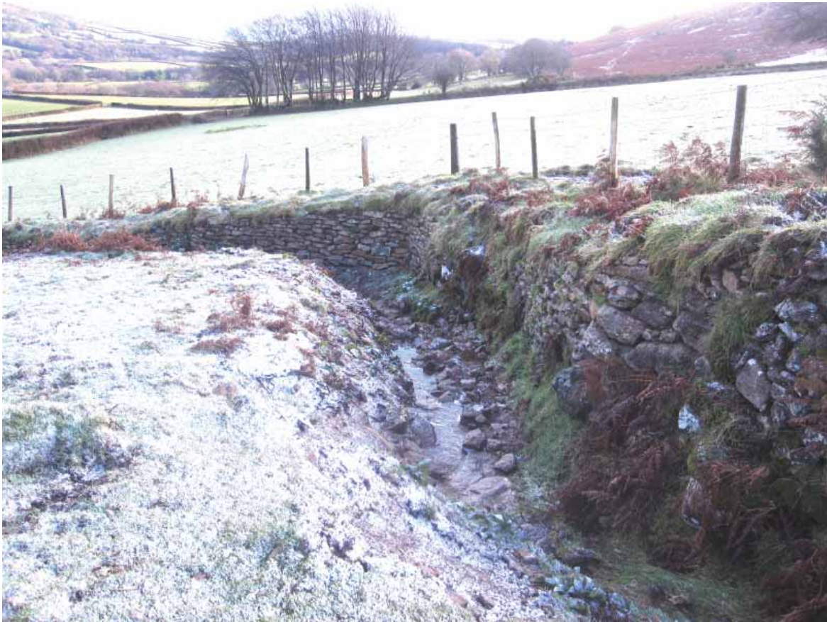
Fig. 8. Part of section CD2, which is almost below ground level. Note both repaired and untouched sections and the watercourse well away from the base of the wall.
