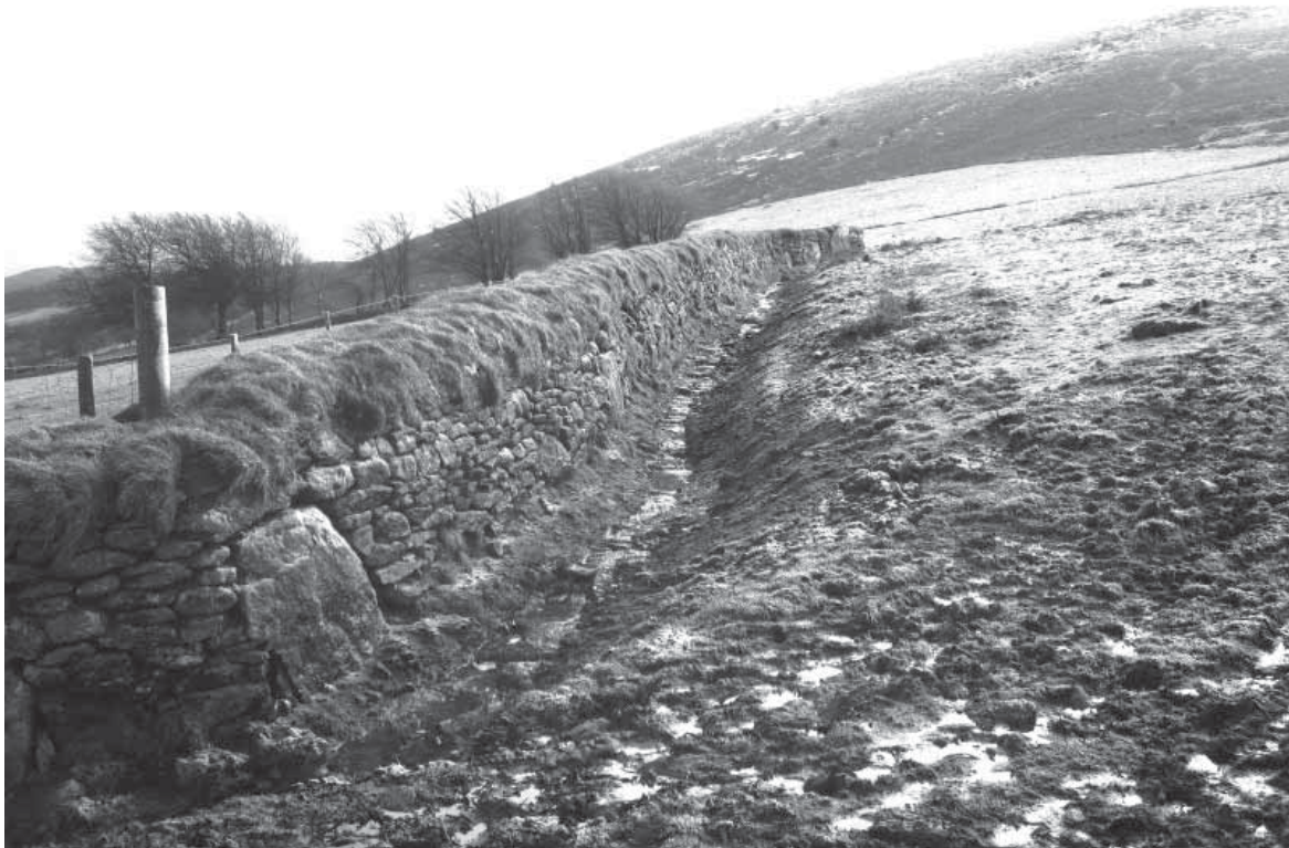
Fig. 1. Section CD3 after repairs.
