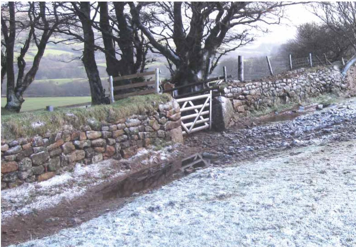
Fig. 9. Gateway on to the moorland within the corn ditch. Note completed section to left, ditch re-dug, wall re-turfed and fence moved to bottom of bank, but post and rails erected against sheep that might climb the wall and jump down behind the gate. The wall to the right has been repaired, but the old unsightly fence is still in place on top.
