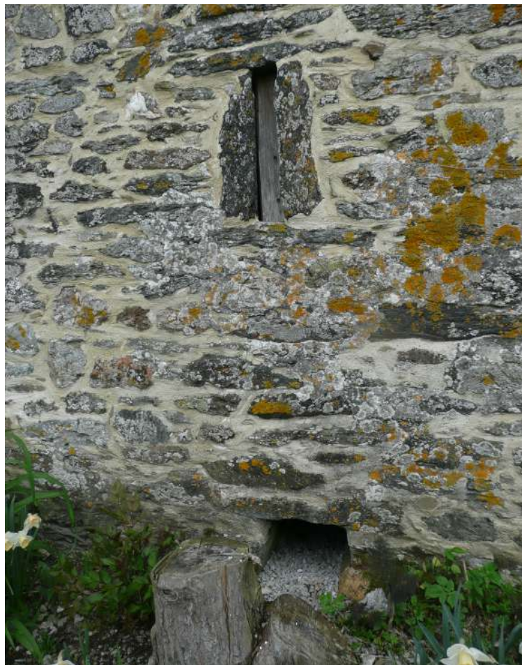
Figure 14. The lower end is still identifiable as a longhouse shippon from the large central drain hole. (Jenny Sanders). The drawing (right) shows two phases of drain in the shippon end to the right, one centrally located and one off-centre. (JRL Thorp, Keystone, 1990).
