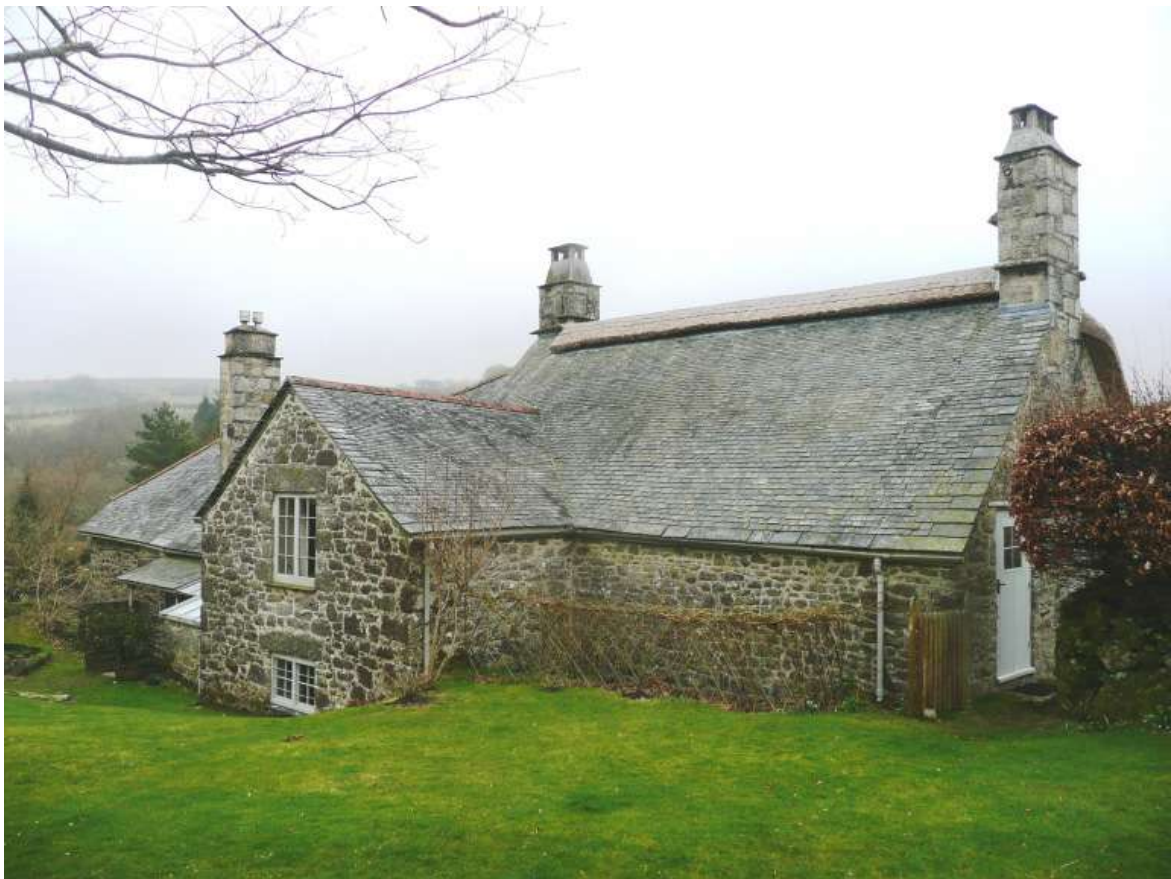
Figure 2. The rear of Bowden in 1995 and 2011. The 20th century windows have been replaced with small-pane casements. (Jenny Sanders).
