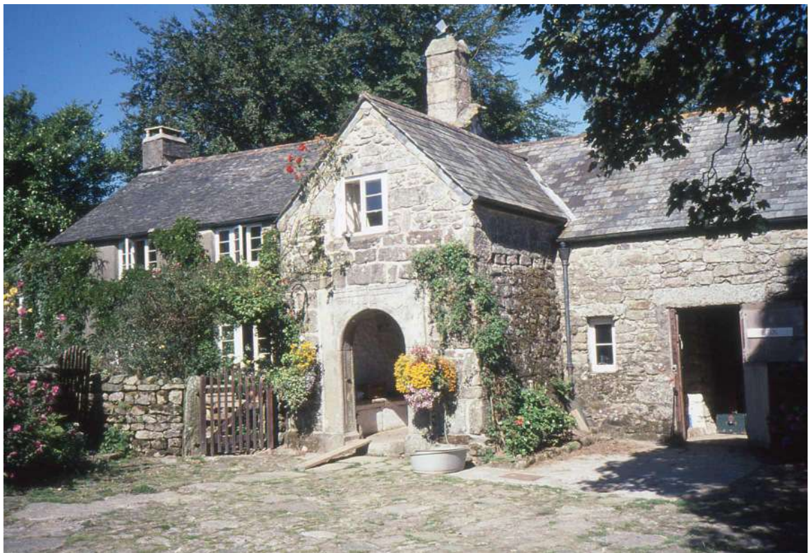
Figure 5. The front elevation of the house in 1975 and 2002 (and see front cover, photographed by the late Elizabeth Gawne). The revived granite paving to the yard is an important part of the architecture of the farmhouse. (Jenny Sanders).
