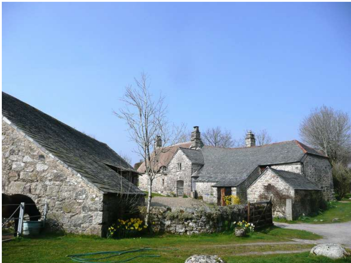
Figure 1. The front elevation of Bowden in 1995 and 2011. The slurried slate roof has been replaced and renewed using small graduated slates and without losing the bow in the ridge that indicates the great age of the building. (Jenny Sanders).
