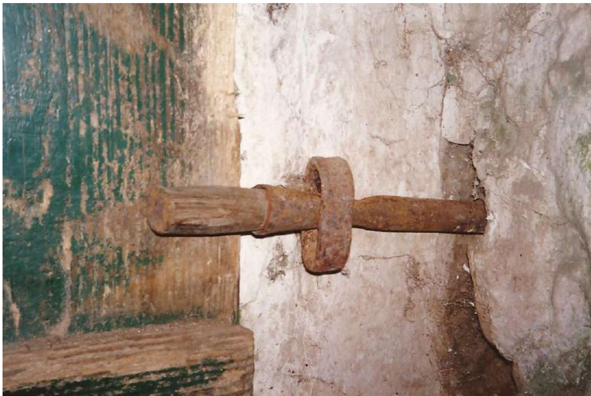
Figure 6. The simple blacksmith-made iron and wooden door bolt (still in use!) is the kind of vernacular feature that is easily lost in a restoration. (Jenny Sanders).
