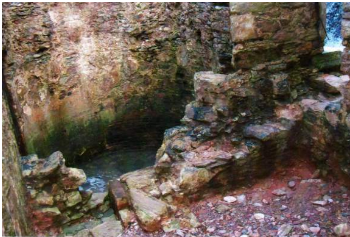
Plate 9. Steps leading down to the brick lined bath.
