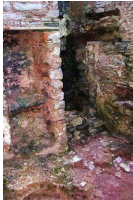
Plate 10. The fire place on the wall opposite the bath. A fire place was part of a bath house so the bather could warm up after a dip and then enjoy the “pleasure” room above.
