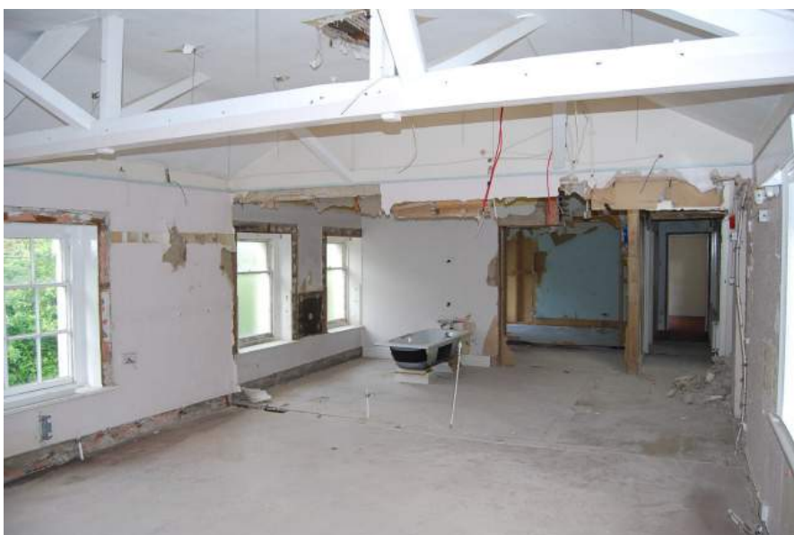
Plate 4. Typical internal view, showing surviving roof construction.
