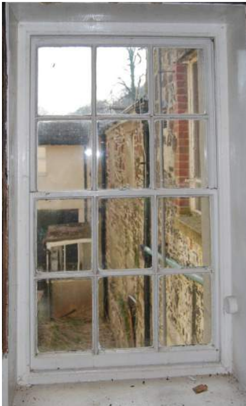
Plate 6. Surviving sash window to light the stairs in the Central Rear Wing (D1).
