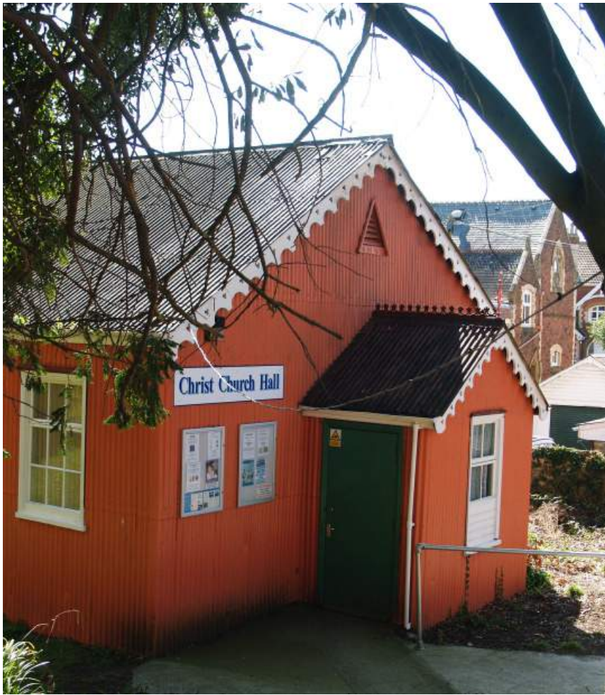
Plate 10. Christ Church, Torquay Road, Paignton. Temporary church erected before the stone church and then re-used as church hall.
