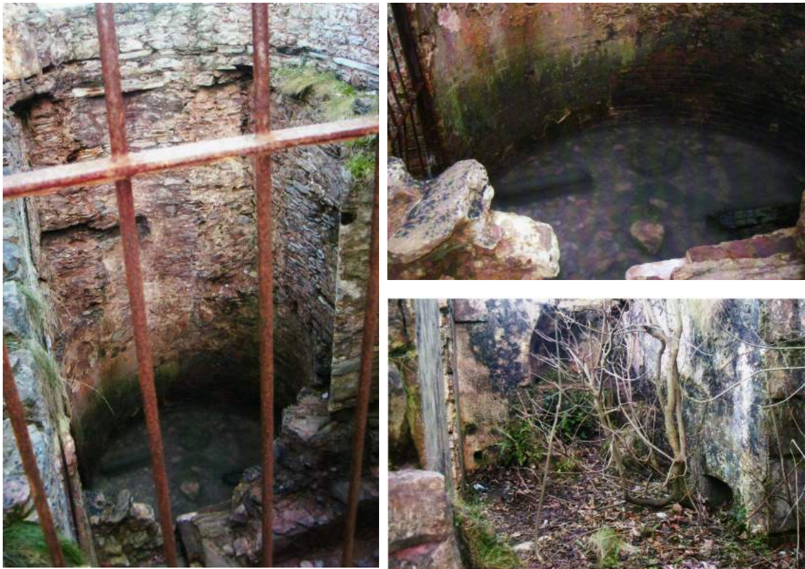
Plates 11, 12 & 13. The bath was filled with sea water at high tide. There was a copper cauldron which heated water. Lady Churston's butler was responsible for lighting the fire and adding the heated sea water to the bath.
