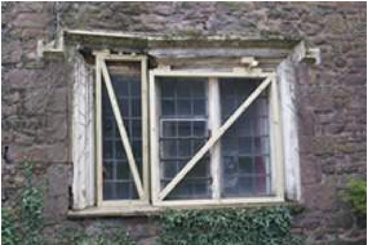
Plate 4. Some of the windows on the front elevation are in very poor condition.
