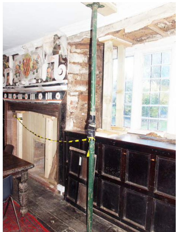
Plate 6. Propping as a temporary solution to problems with the west wall of the hall.
