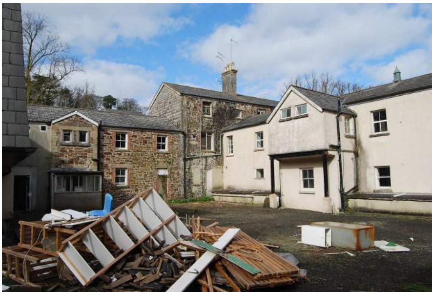
Plate 3. The south-eastern rear yard of Okehampton Workhouse, looking west shortly before it was demolished. The taller block was the Hub, or Master's House.
