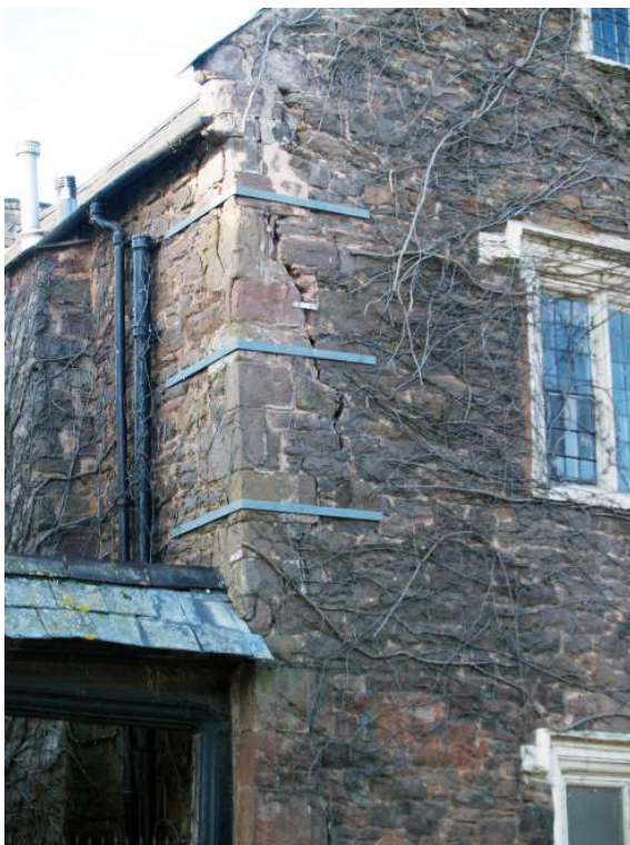
Plate 5. Temporary repairs have been undertaken to secure the fabric in advance of much needed capital works.
